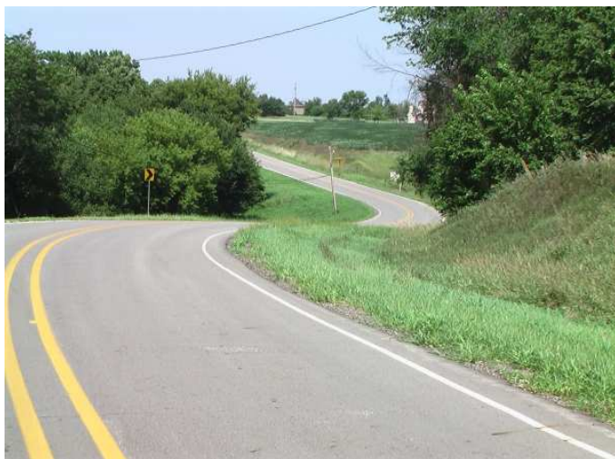
Dangerous Curvy section on Frisk Drive
